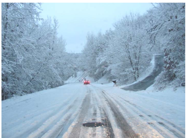
to adjust to road and shoulder conditions
